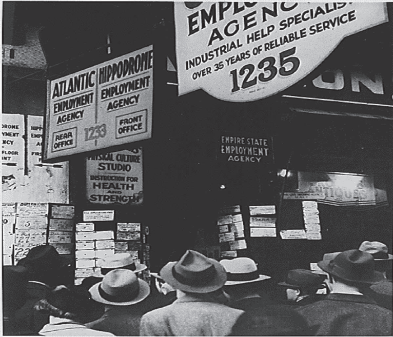
(Franklin D. Roosevelt Library, courtesy of the National Archives and Records Administration).
